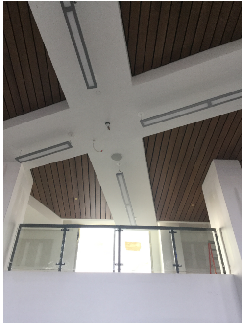
Fitness Center Ceiling
